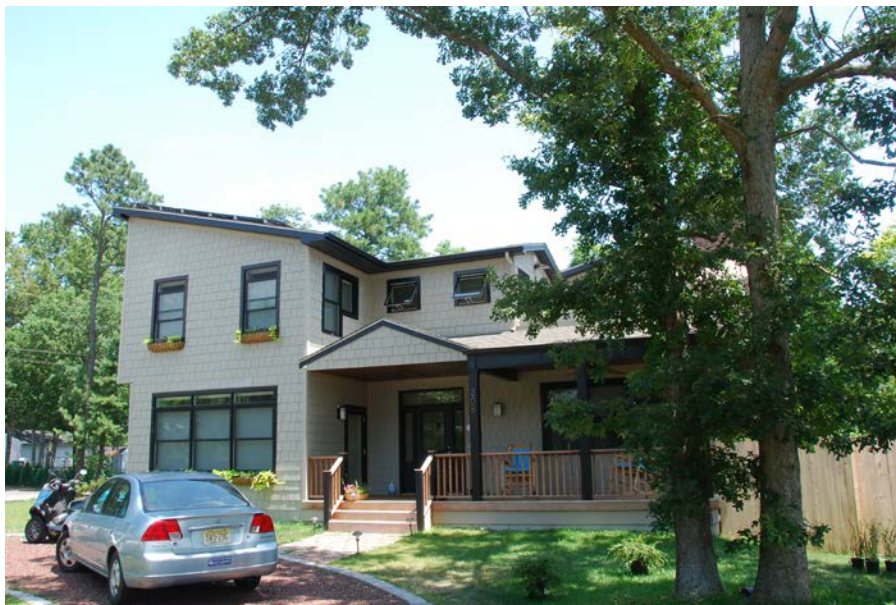
exterior - west facade
